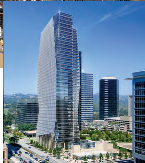
A rendering of the under-construction Century City Center (courtesy of Johnson Fain)
